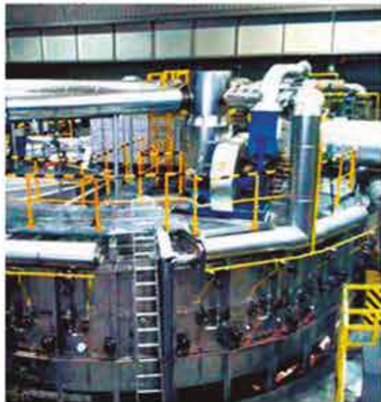
Ring heating furnace
